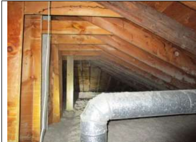
Location: 347 Depot St Jamaica, VT Photo Taken By: Richard Lalancette, P.E. IMG: 224 Description: Attic over original building
