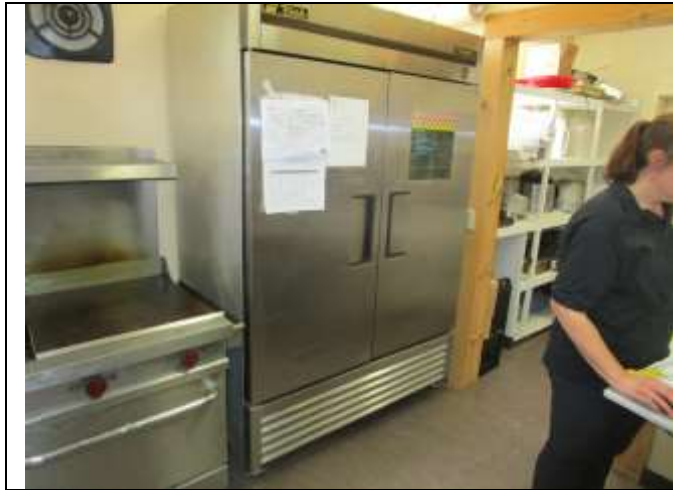
Location: 347 Depot St Jamaica, VT Photo Taken By: Richard Lalancette, P.E. IMG: 202 Description: Kitchen refrigerator
