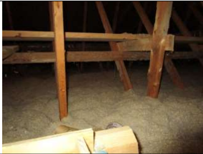
Location: 347 Depot St Jamaica, VT Photo Taken By: Richard Lalancette, P.E. IMG: 219 Description: Attic space over original building
