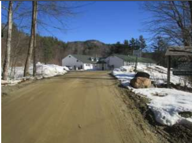
Location: 347 Depot St Jamaica, VT Photo Taken By: Richard Lalancette, P.E. IMG: 122 Description: Exit driveway from property
