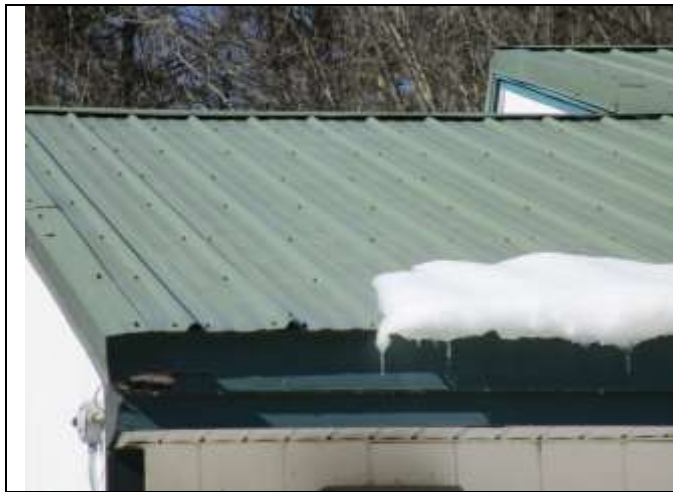
Location: 347 Depot St Jamaica, VT Photo Taken By: Richard Lalancette, P.E. IMG: 174 Description: Roof surface
