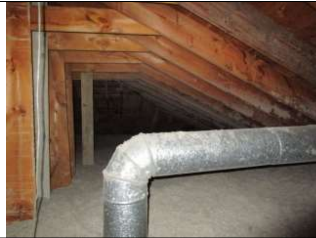
Location: 347 Depot St Jamaica, VT Photo Taken By: Richard Lalancette, P.E. IMG: 223 Description: Attic over original building
