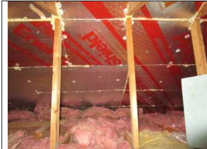
Location: 347 Depot St Jamaica, VT Photo Taken By: Richard Lalancette, P.E. IMG: 216 Description: Attic space
