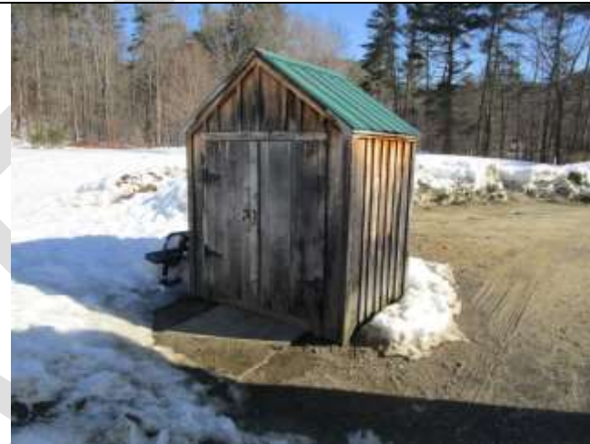
Location: 347 Depot St Jamaica, VT Photo Taken By: Richard Lalancette, P.E. IMG: 128 Description: Small shed
