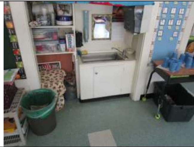
Location: 347 Depot St Jamaica, VT Photo Taken By: Richard Lalancette, P.E. IMG: 211 Description: Cabinetry in older classroom
