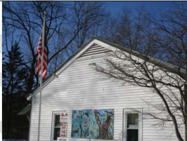
Location: 347 Depot St Jamaica, VT Photo Taken By: Richard Lalancette, P.E. IMG: 132 Description: Typical building mounted lighting
