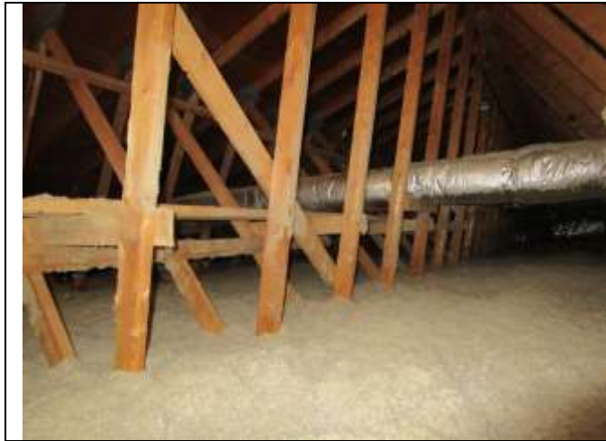
Location: 347 Depot St Jamaica, VT Photo Taken By: Richard Lalancette, P.E. IMG: 222 Description: Attic over original building
