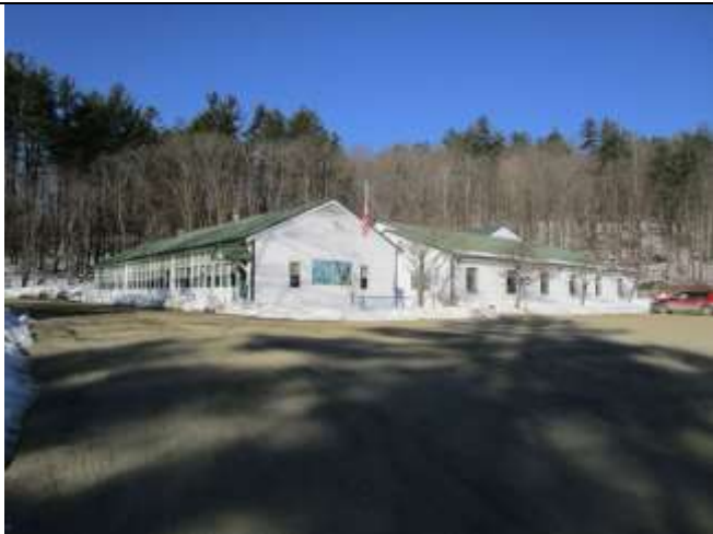
Location: 347 Depot St Jamaica, VT Photo Taken By: Richard Lalancette, P.E. IMG: 118 Description: Left front of building
