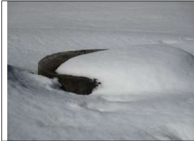
Location: 347 Depot St Jamaica, VT Photo Taken By: Richard Lalancette, P.E. IMG: 125 Description: Well at rear of building
