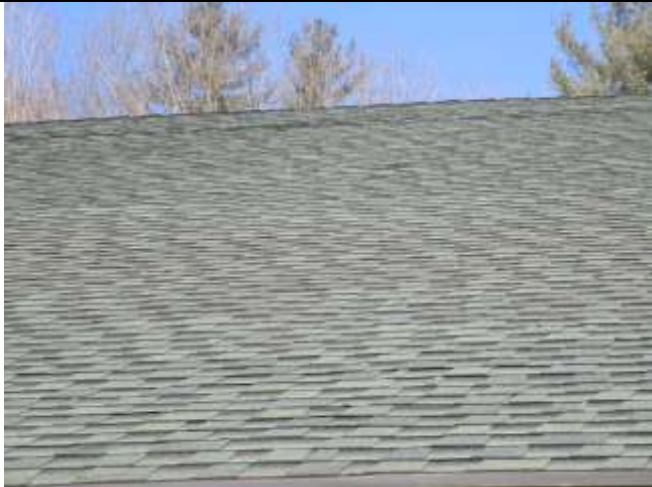
Location: 347 Depot St Jamaica, VT Photo Taken By: Richard Lalancette, P.E. IMG: 184 Description: Asphalt shingle roof surfacing
