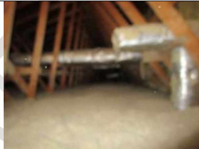
Location: 347 Depot St Jamaica, VT Photo Taken By: Richard Lalancette, P.E. IMG: 217 Description: Attic space
