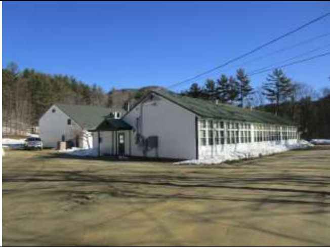
Location: 347 Depot St Jamaica, VT Photo Taken By: Richard Lalancette, P.E. IMG: 120 Description: Left rear of building
