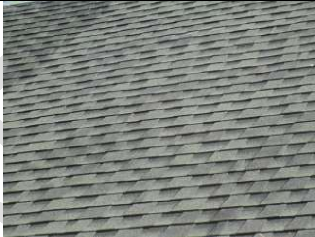
Location: 347 Depot St Jamaica, VT Photo Taken By: Richard Lalancette, P.E. IMG: 185 Description: Asphalt shingle roof surfacing.
