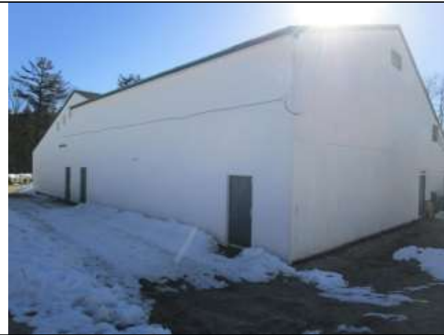
Location: 347 Depot St Jamaica, VT Photo Taken By: Richard Lalancette, P.E. IMG: 126 Description: Right side of multi- purpose room
