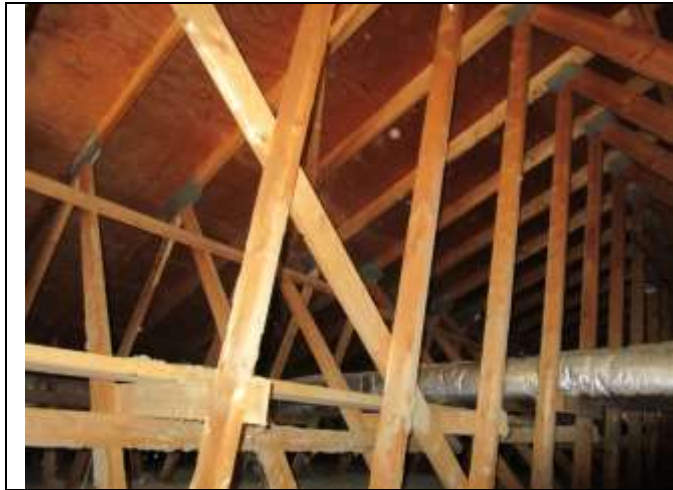
Location: 347 Depot St Jamaica, VT Photo Taken By: Richard Lalancette, P.E. IMG: 218 Description: Attic space with trusses
