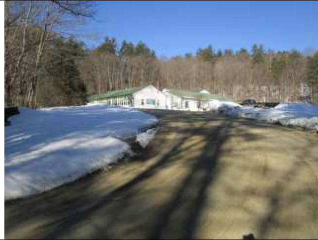
Location: 347 Depot St Jamaica, VT Photo Taken By: Richard Lalancette, P.E. IMG: 117 Description: Gravel driveway to building
