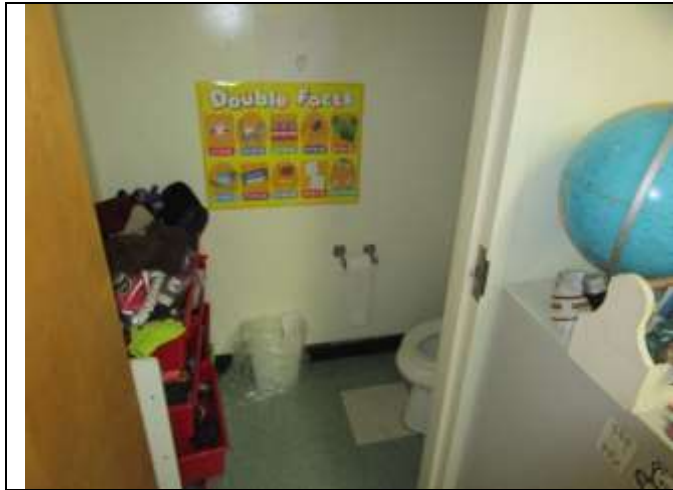
Location: 347 Depot St Jamaica, VT Photo Taken By: Richard Lalancette, P.E. IMG: 210 Description: Typical toilet in classroom
