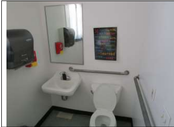
Location: 347 Depot St Jamaica, VT Photo Taken By: Richard Lalancette, P.E. IMG: 214 Description: Hallway girl's room
