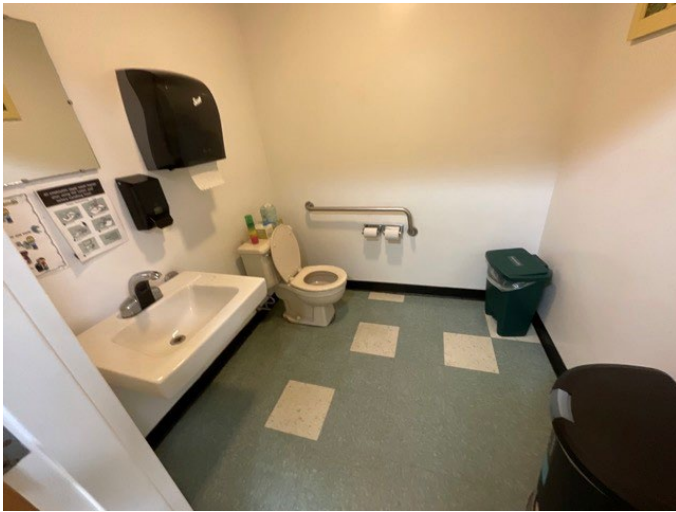
9 - TOILET STALL OVERVIEW
