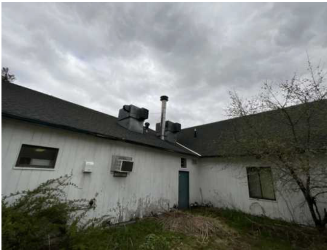
9 - SECONDARY ROOF ASPHALT SHINGLES
