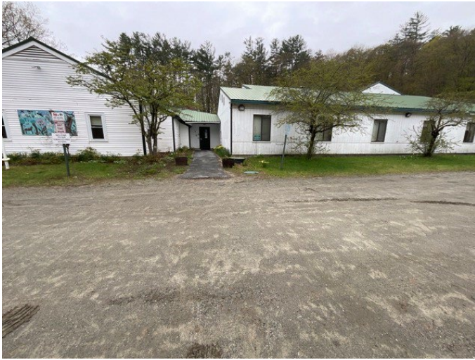
1 - OVERVIEW OF ACCESSIBLE PARKING AREA
