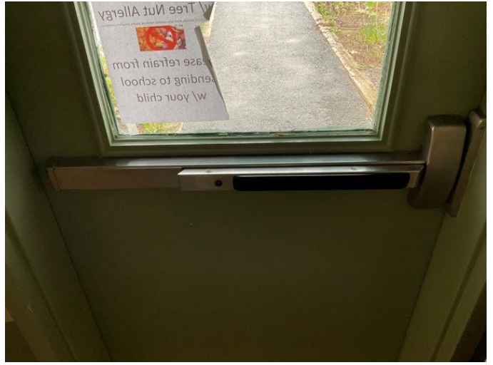
8 - HARDWARE, STAIR RAILS
