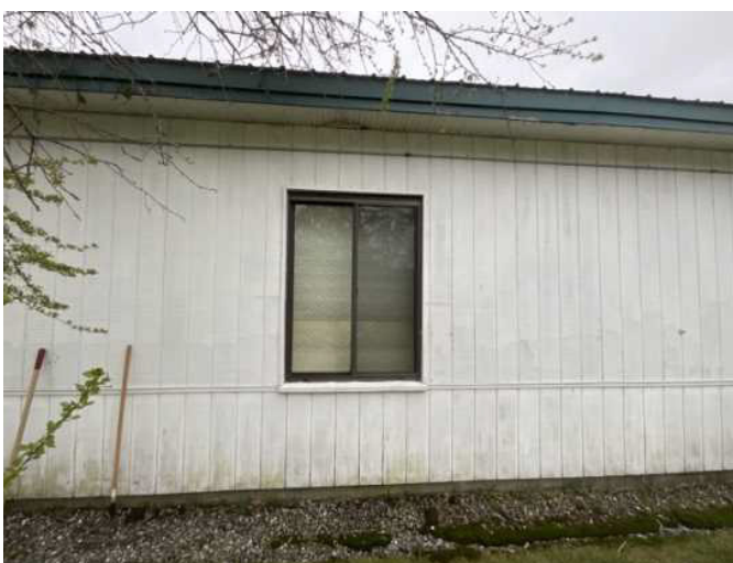
5 - BUILDING FACADE WOOD SIDING
