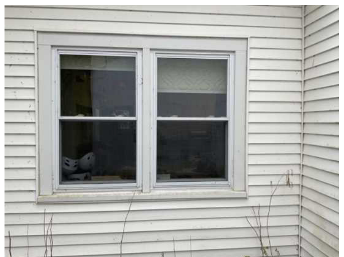
6 - BUILDING FACADE VINYL SIDING
