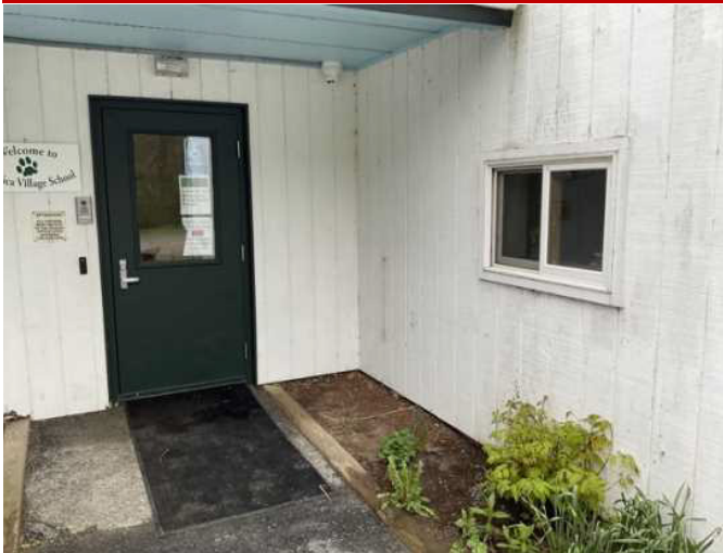
7 - MAIN ENTRANCE TO SCHOOL
