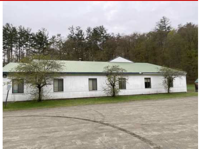
8 - PRIMARY METAL ROOF OVERVIEW
